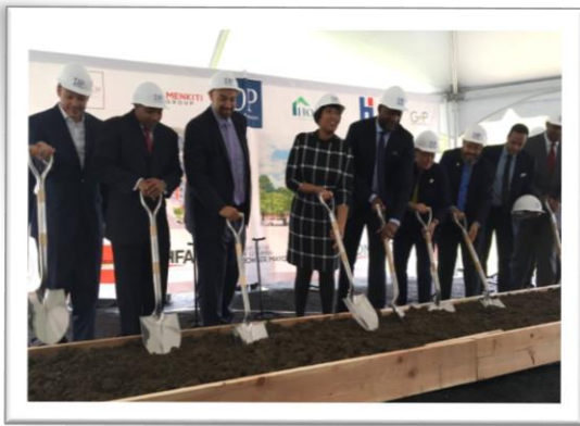
Mayor Bowser with the Capitol Vista development team breaking ground on Capitol Vista.
